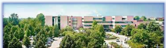
Humanitas Research Hospital, Italy
